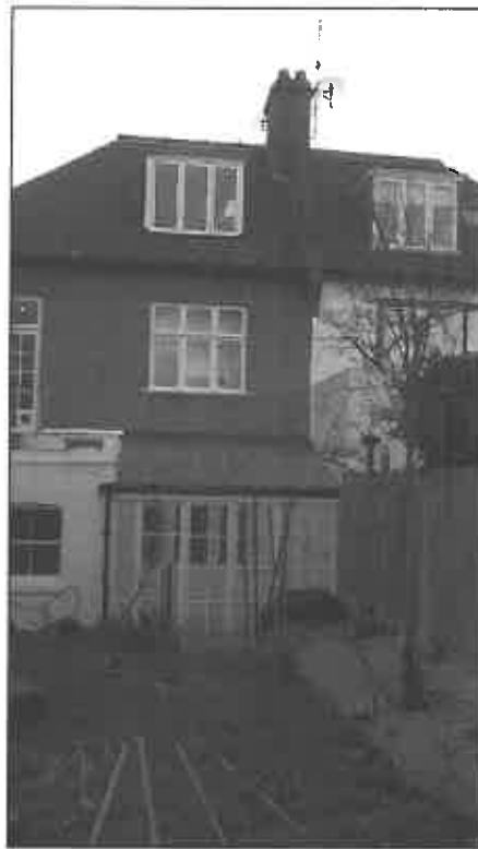
Photo 5 - View of rear of house
