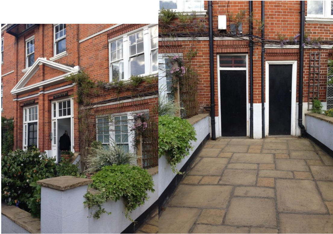
Photograph Three : (Left) residential entry to flats above (Wentworth Mansions), (right) the existing rear doors to the commercial ground floor units.
