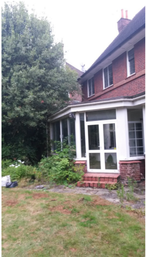
Looking northwards across rear elevation
