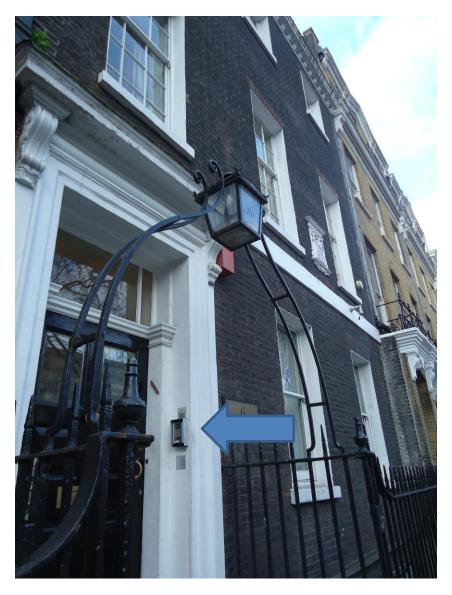
New door entry system to be installed in the same location as existing shown. There will be no security alarms, cameras, additional lighting or display screens etc. New external grilles at basement front door are shown in accompanying dwgs.
