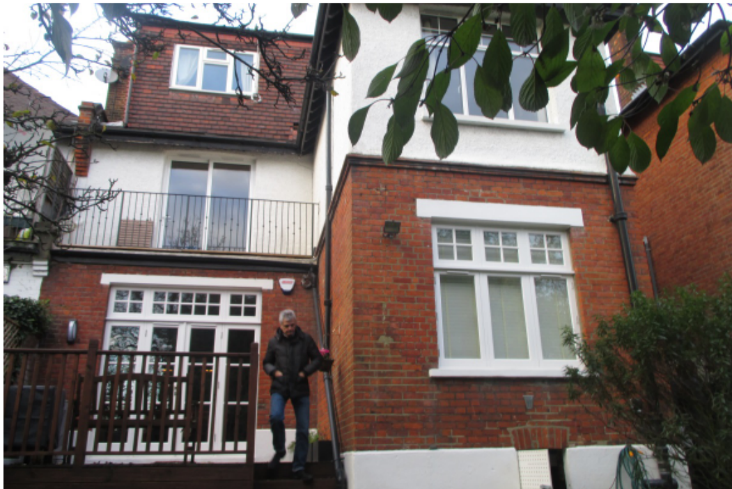
View of rear of house
