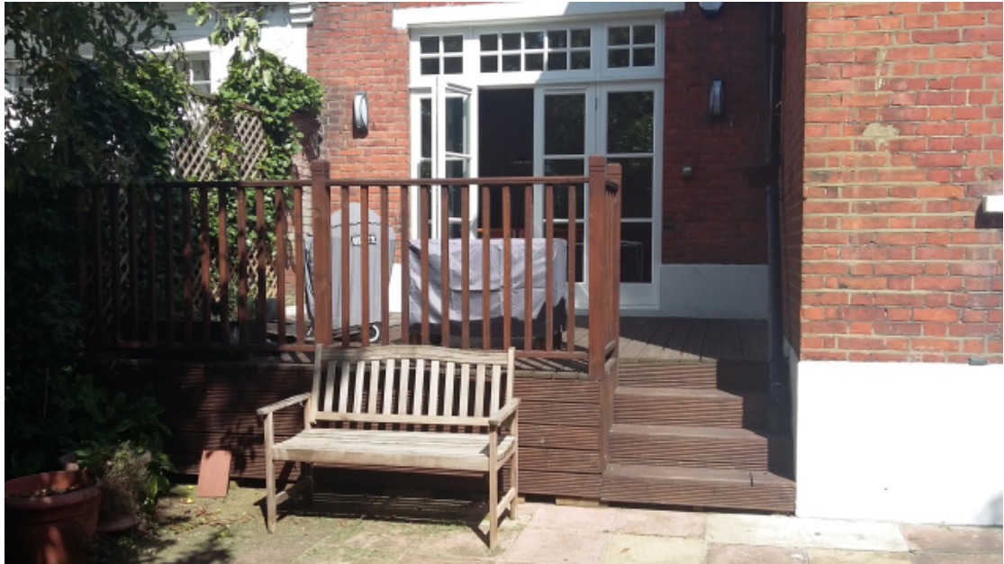
View of decking area
