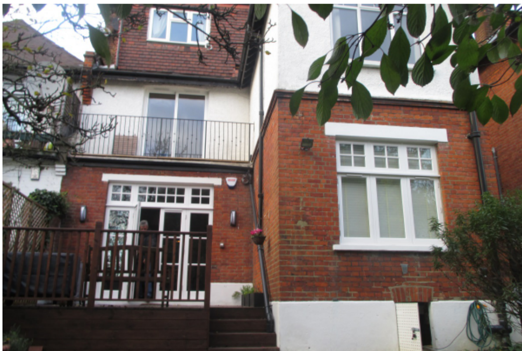
View of rear of house
