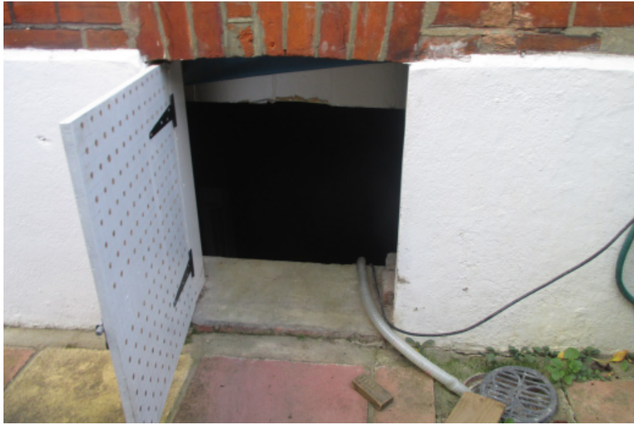
Entrance to existing void below building
