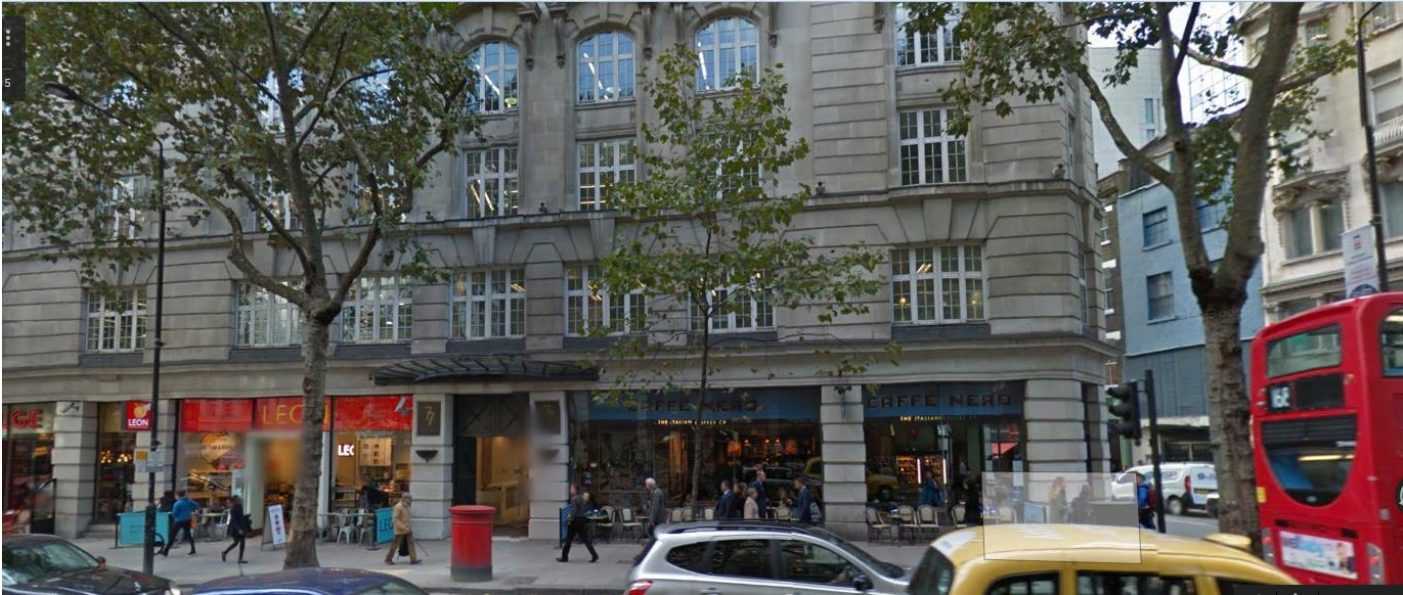
Photo 1- Existing Front Elevation
