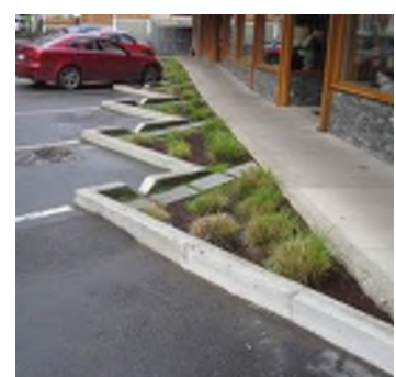
Rain gardens in Toronto taking surface water from car park and pedestrian areas (Photos: Dusty Gedge)
