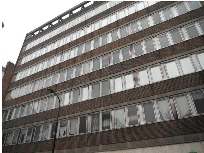
Photograph 1 Building 1 (Arthur Stanley House).
