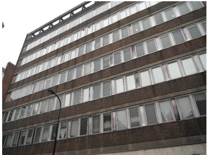
Photograph 1 Building 1 (Arthur Stanley House).
