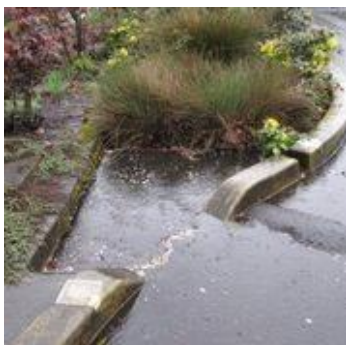
Rain gardens in Toronto taking surface water from car park and pedestrian areas (Photos: Dusty Gedge)
