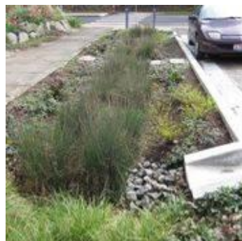
Rain gardens in Toronto taking surface water from car park and pedestrian areas (Photos: Dusty Gedge)
