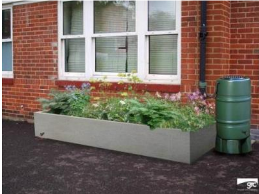
Rain garden planter providing storm water/SuDS feature and amenity/visual value (Image: The Green Roof Consultancy)
