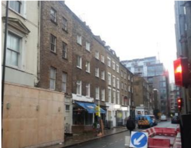
Georgian terraces on south side of Tottenham Street with later facades. Listed No 39 on near corner of Goodge Place
