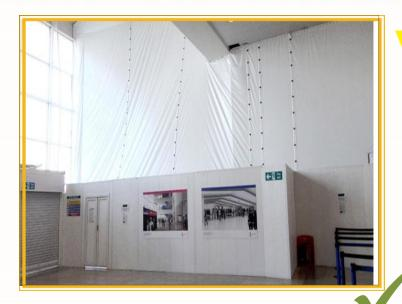
Flexiscreen temporary screens and hoardings provide a dust-tight seal to screen processes and work areas. Ideal for live environments providing minimal disruption to the public and occupiers of buildings.
