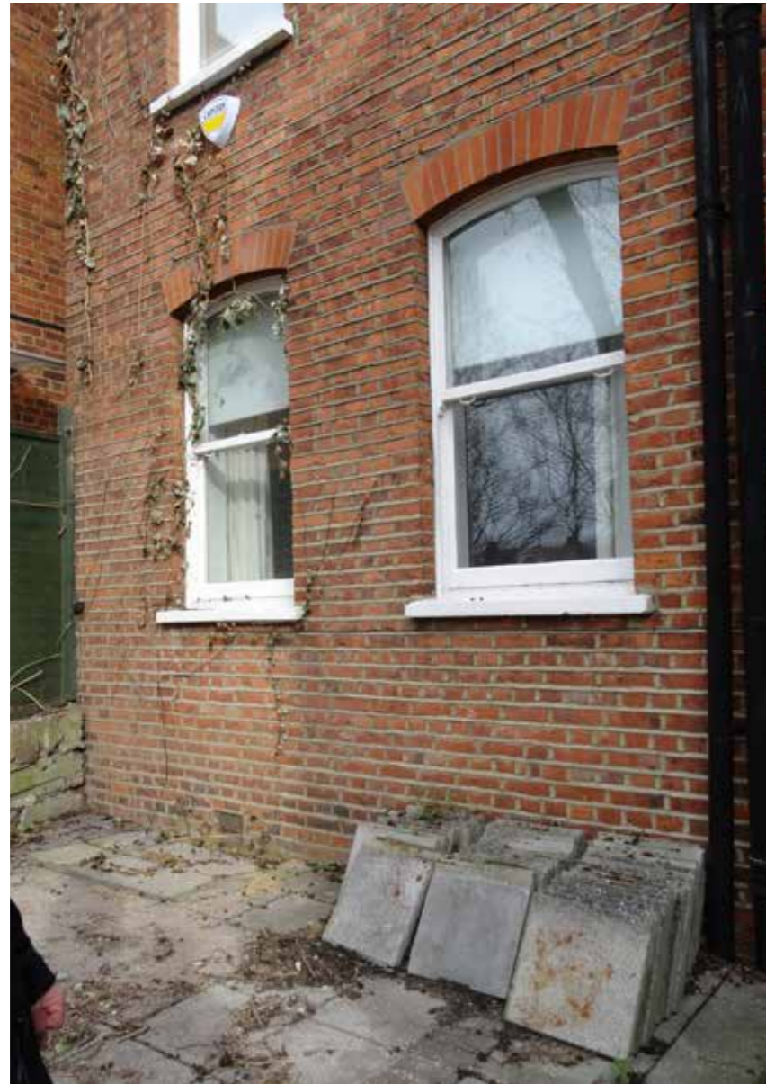
View of Rear Fenestration
