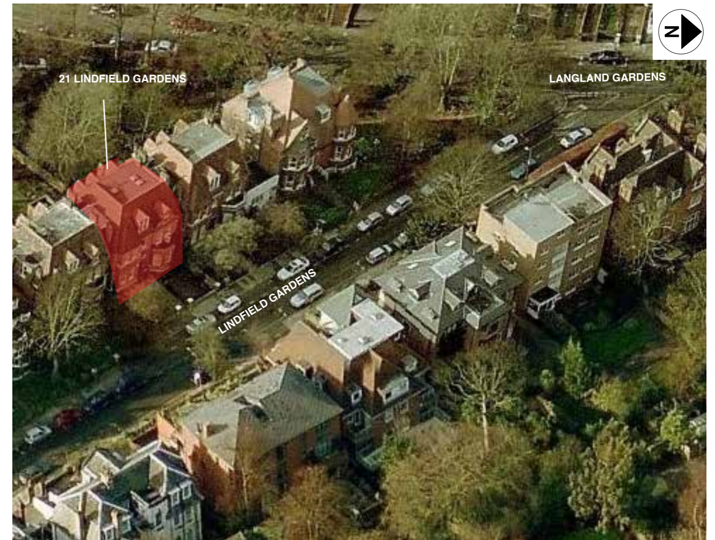
Aerial Photograph Looking West
