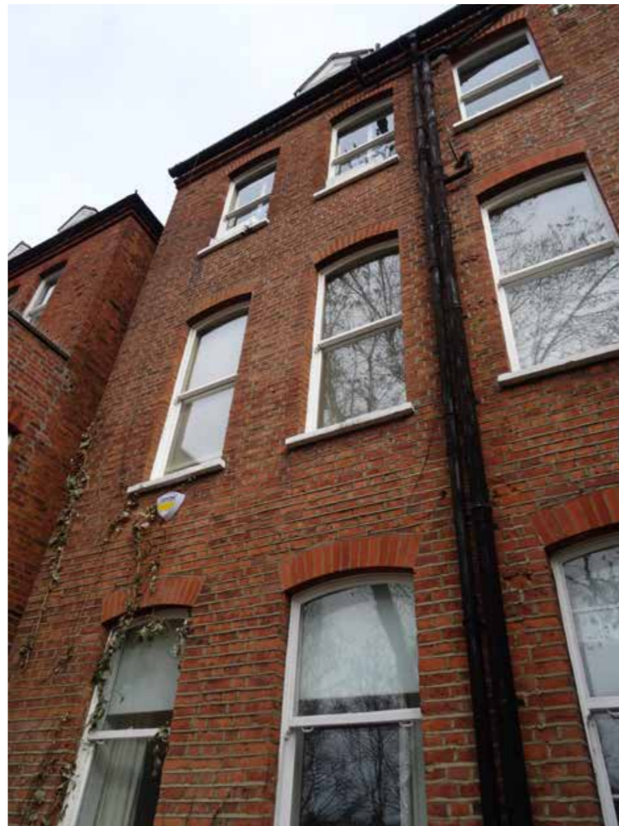
View of Rear Elevation
