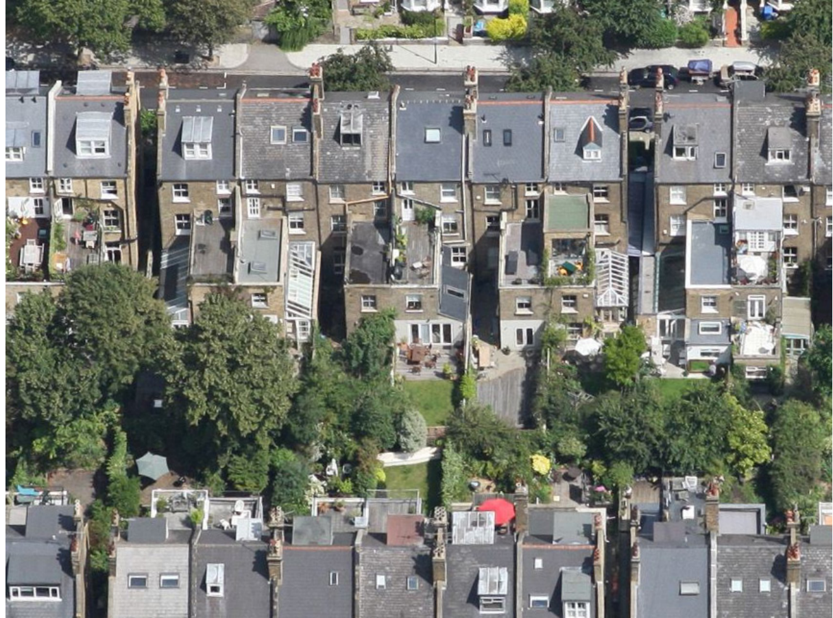
Aerial View of Existing
