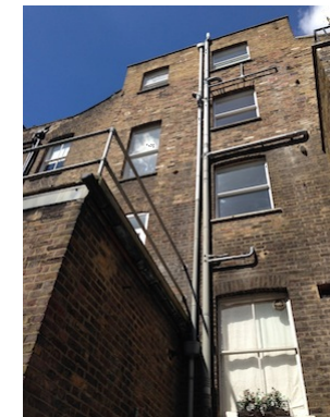
Photo 1 of existing rear elevation
