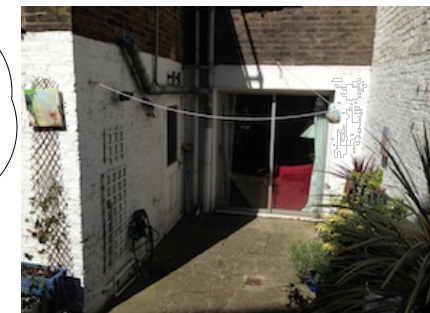
Photo 3 of existing rear elevation
