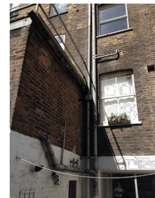
Photo 2 of existing rear elevation
