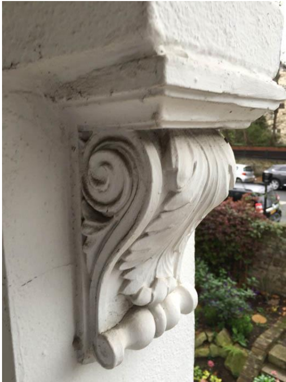
Figure 5: (Existing) Corbels in the entrance porch of 56 are very different from the originals
