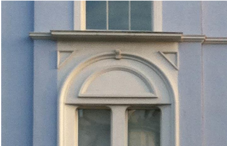
Figure 1: (Existing) Main bay of 56 was rendered flat with sections of pre-cast moulding applied to the surface. Decorative cast iron panel is missing from second floor window sill
