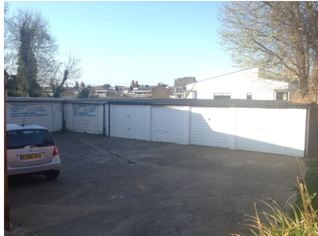
02 Line of garages with 202 Finchley Road visible behind.
