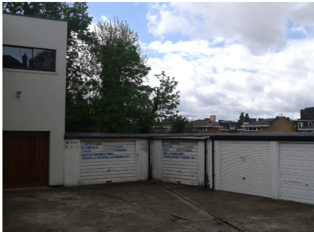
01 New build house and garages.
