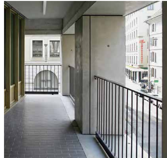
Precedent: Sergison Bates Architects - Urban Housing & Creche, Geneva. Slim profile bespoke metal balustrades with high quality floor finish to amenity spaces
