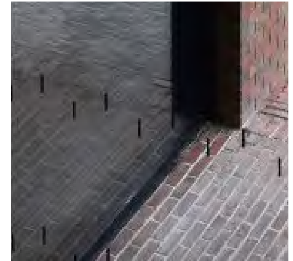
Precedent: Duggan Morris Architects - Yew Tree Lodge. Brick pavior apron at base of brick walls to match the brick used for the buildings
