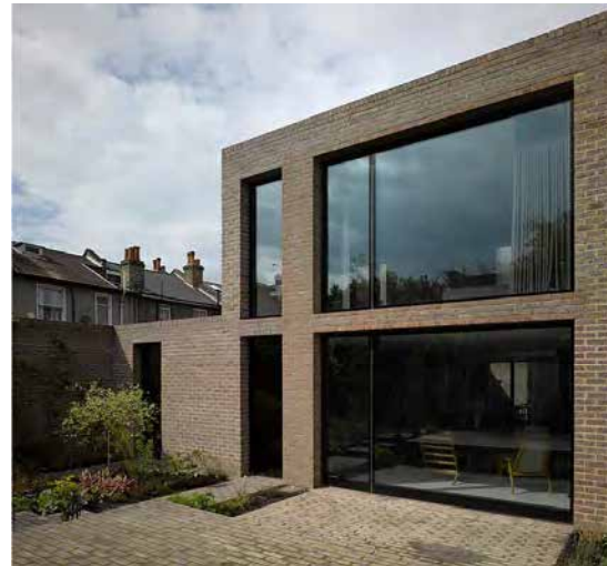
Precedent: Duggan Morris Architects - Kings Grove House. Grey/brown textured brick & header course, with large window recesses
