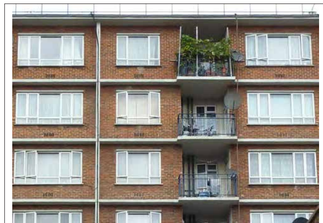
Horizontal concrete decks on Blemundsbury north elevation
