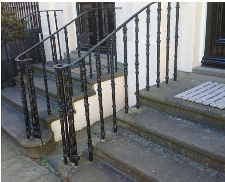
Example image 3 New lightwell step balustrade
