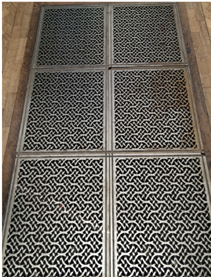
Example image 1 Lightwell grille and stairs ironwork
