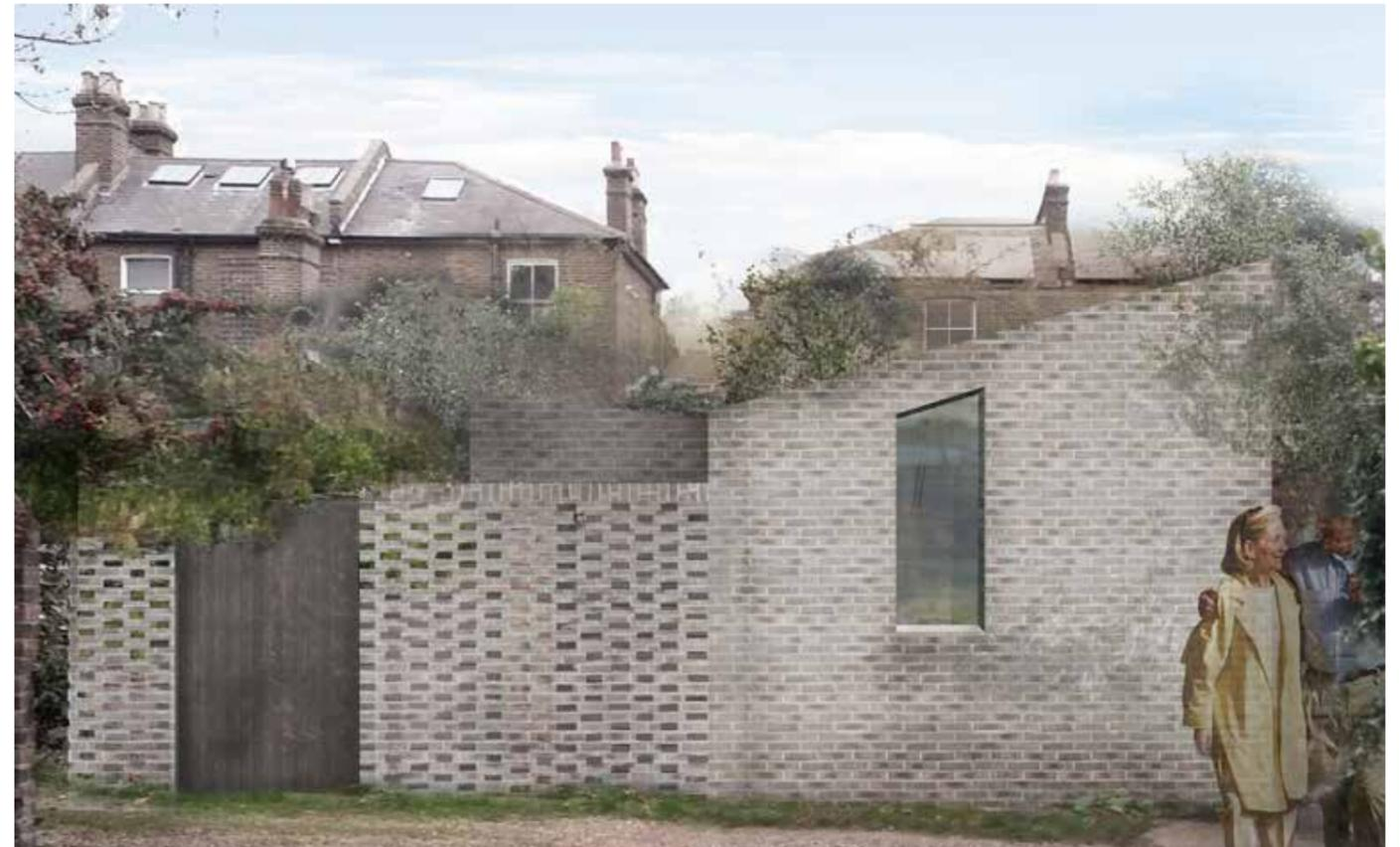
Hit and miss brickwork for the garden walls of the proposed scheme
