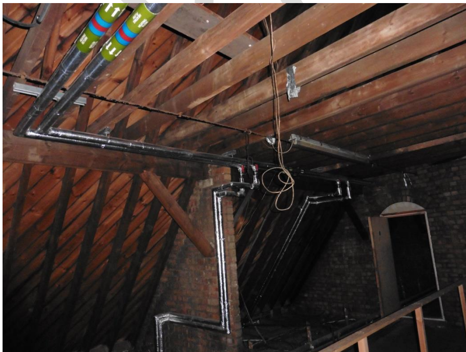
Stub walls supporting propped purlins.
