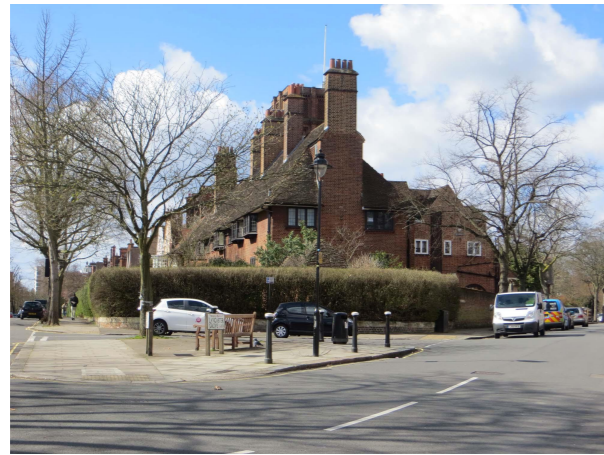
1. View from the east looking west.
