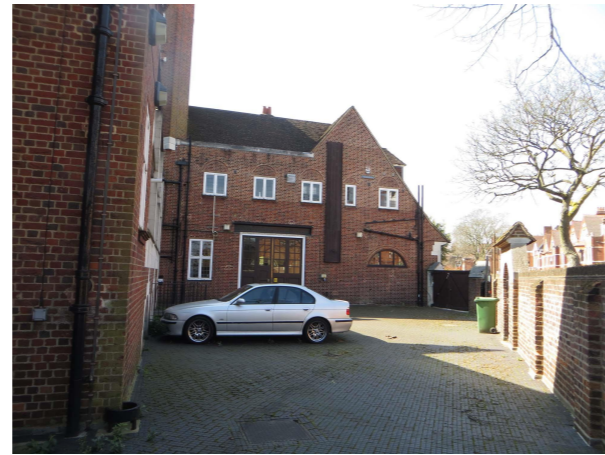
2. View of internal court looking west.
