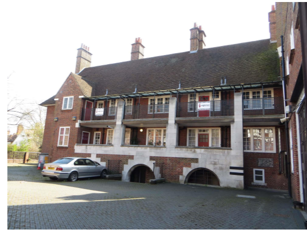
3. View of internal court looking south.
