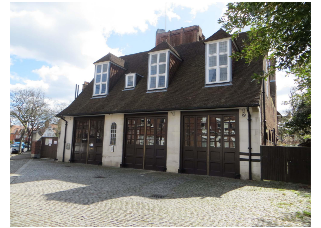
4. View of fire tender bays and court.
