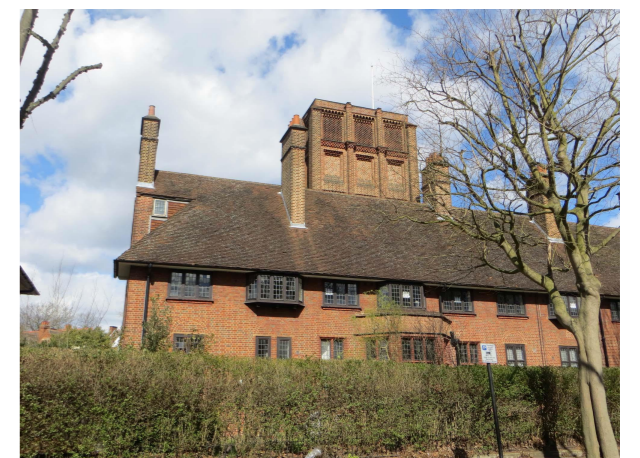
5. View of southwest elevation.
