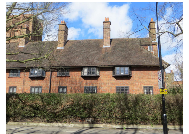
5. View of southeast elevation.
