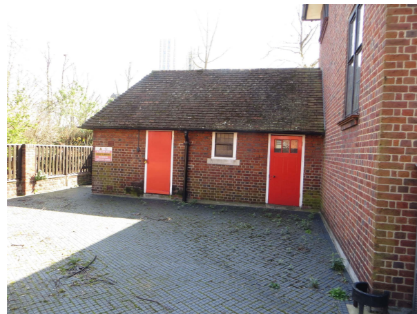
4. View of east store building.
