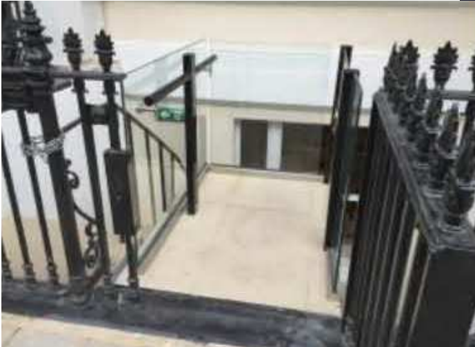
the lift with gate open at pavement level
