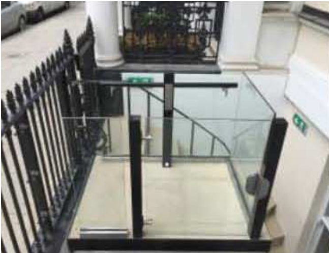
the lift at pavement level
