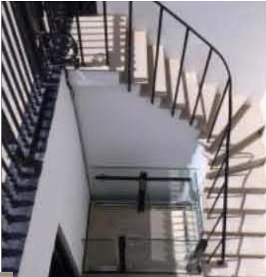
the lift at lower level
