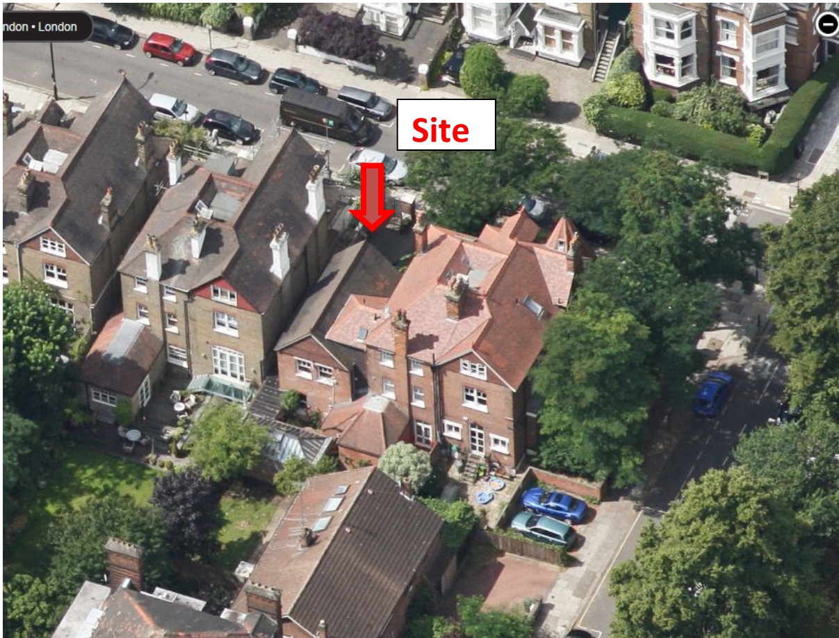
1. Aerial view of the rear of 98A Priory Road
