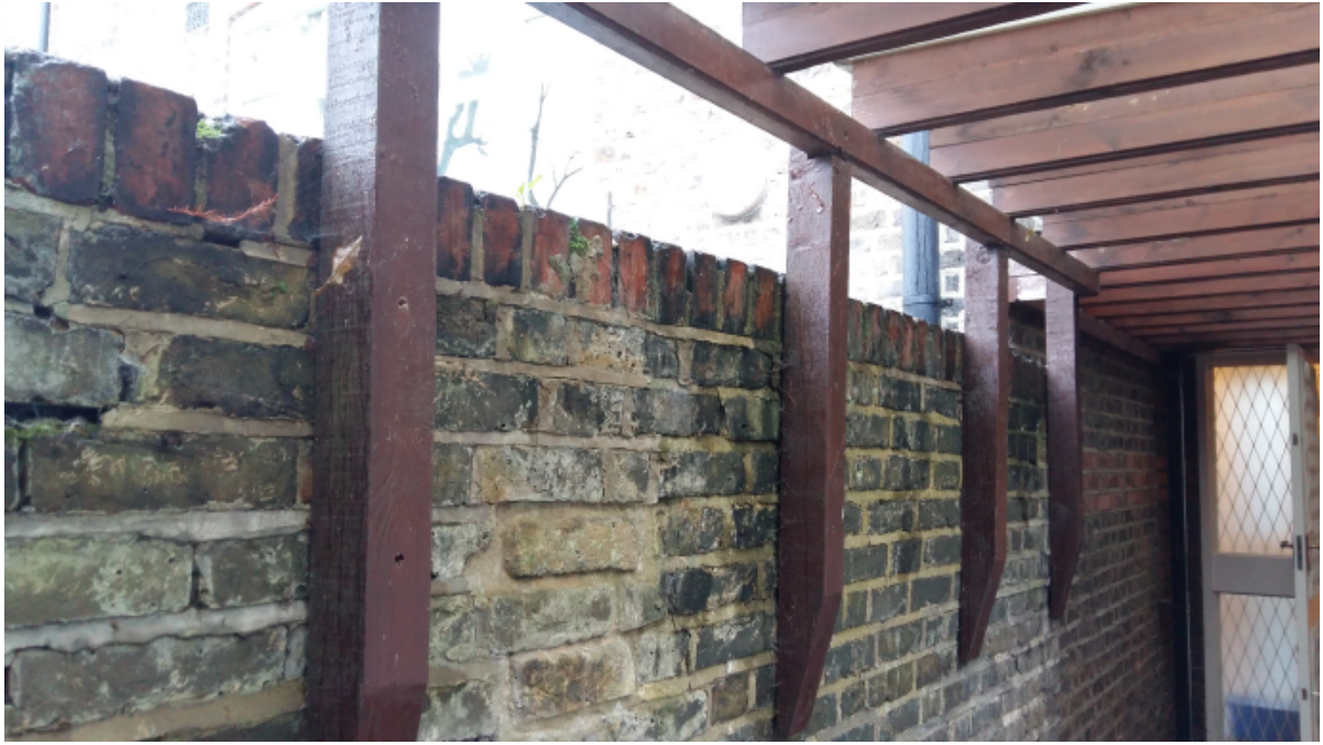
5. Existing pergola structure adjoining no. 96 Priory Road
