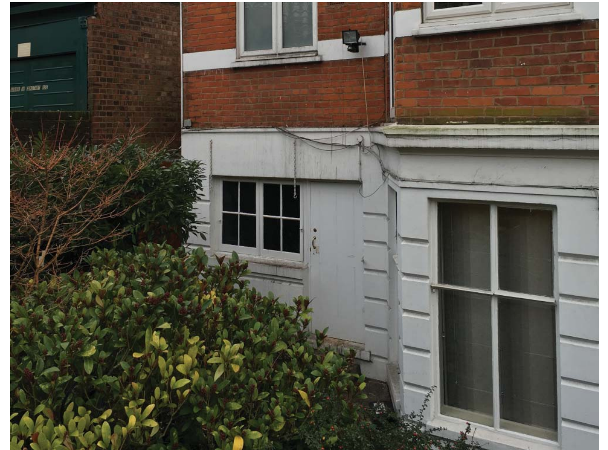
The Existing Street Elevation of the Site
