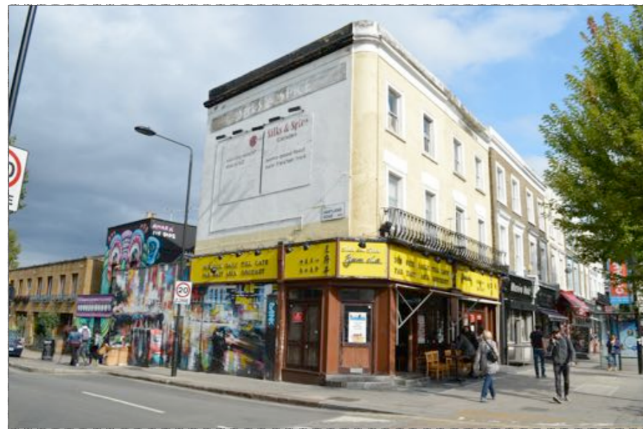
3. EXISTING SITE PHOTO - VIEW FROM WEST CORNER
