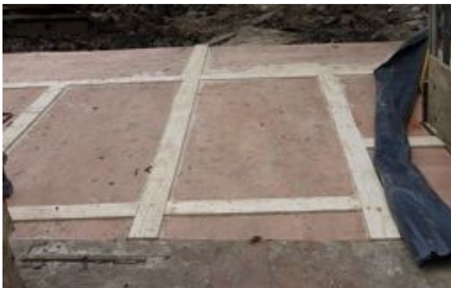
Figure 7. Plywood sheeting used as ground protection.
