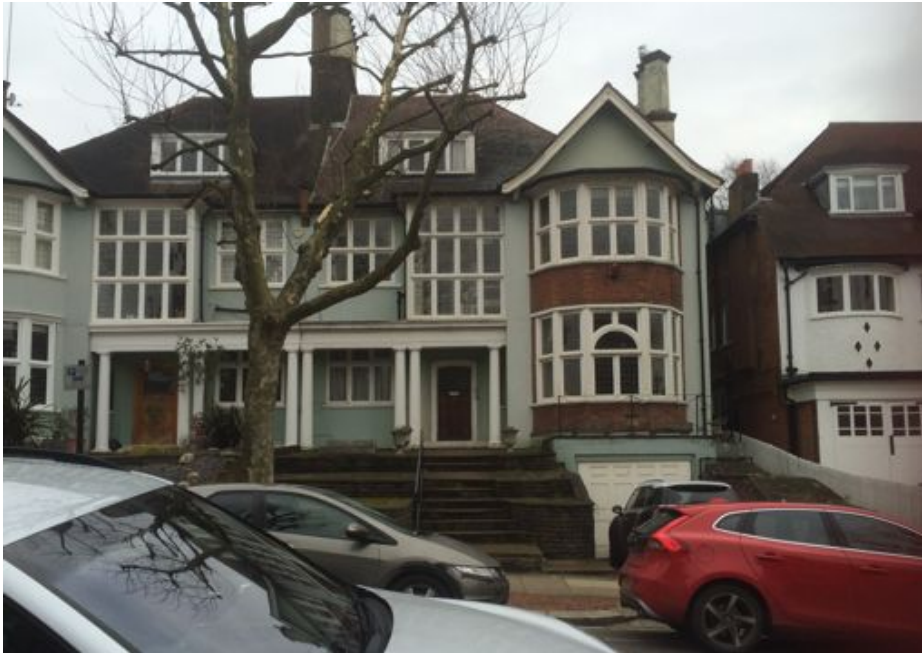
FRONT VIEW OF 14 ROSECROFT AVENUE - HAMPSTEAD – LONDON NW3 5PS
