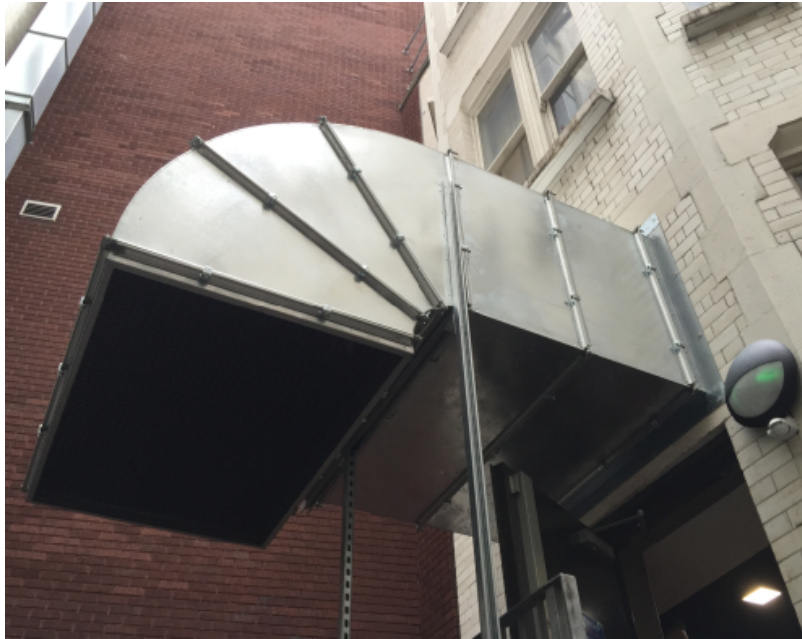
Previous Air Intake Attenuator
