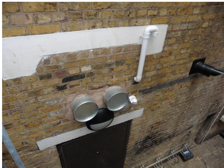
New Capped Boiler Room Vents 1
