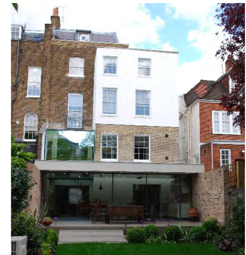
Hamilton Terrace, NW8 - Extension & modernisation of grade II listed terrace house.
