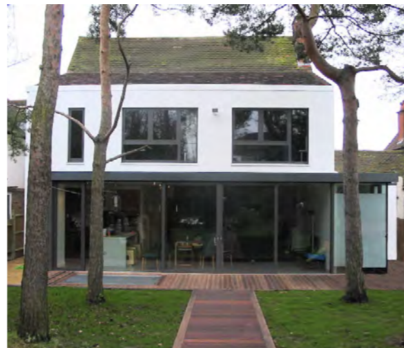
Newcombe Park, NW7 - Extension & modernisation of detached house
