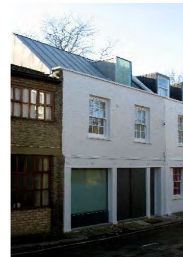
Kingstown Street, NW1 - Partial rebuild & extension to article 4 conservation area mews house
