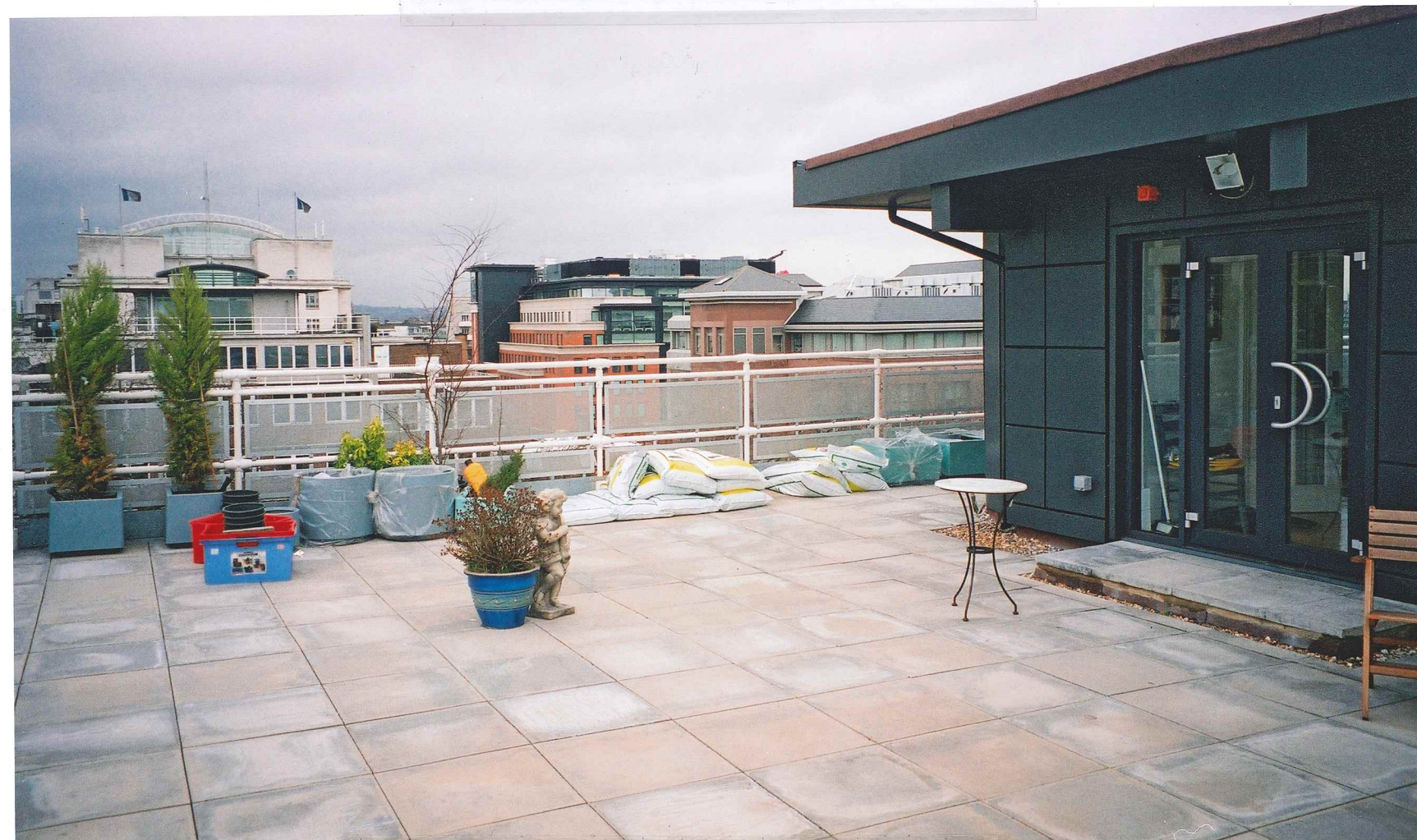
VIEW FROM ROOF TERRACE LOOKING NORTH (across Red Lion Square )
