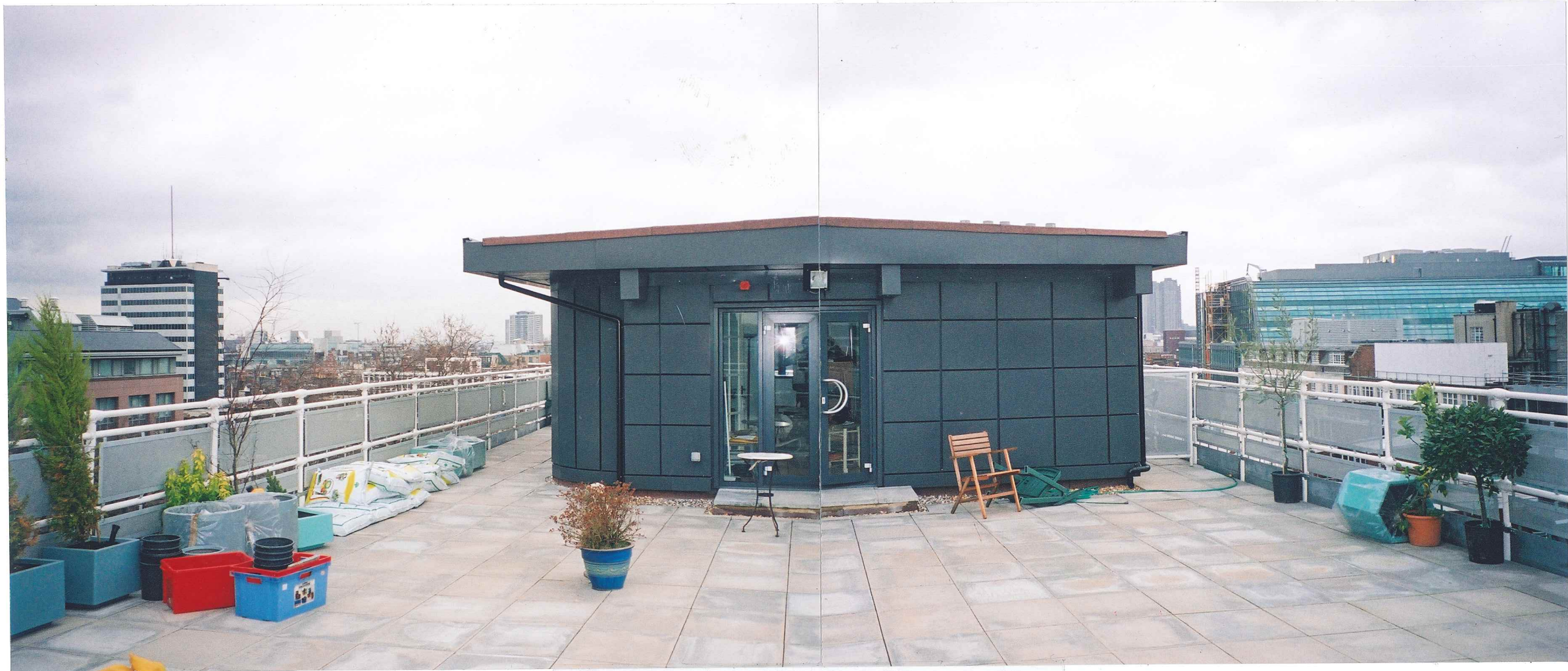
10 RED LION SQUARE – VIEW OF EXISTING 8TH FLOOR (looking east)
