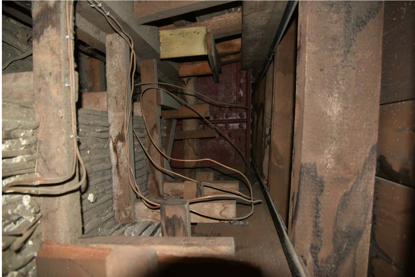
VOID INSIDE THE HATCH
