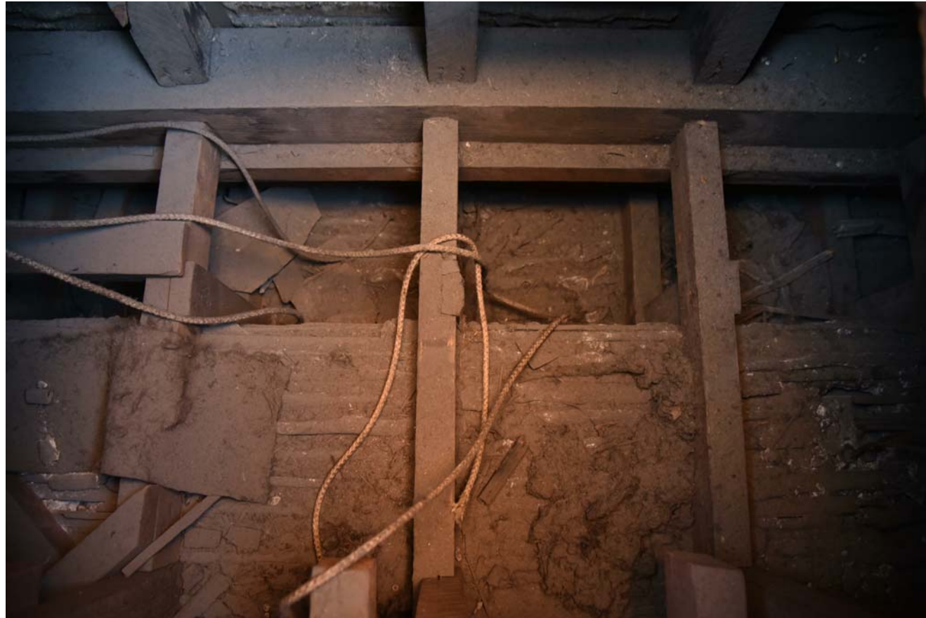
VOID INSIDE THE HATCH
