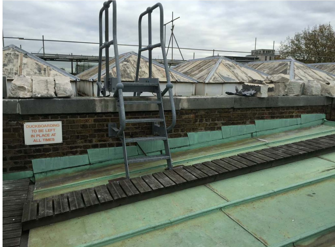
WOODEN WALKWAY TO BE REMOVED
