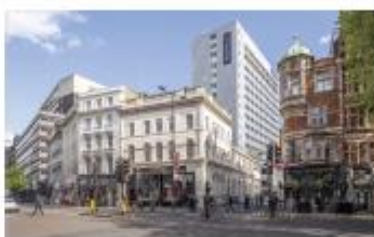
Existing – corner of New Oxford Street & West Central Street
