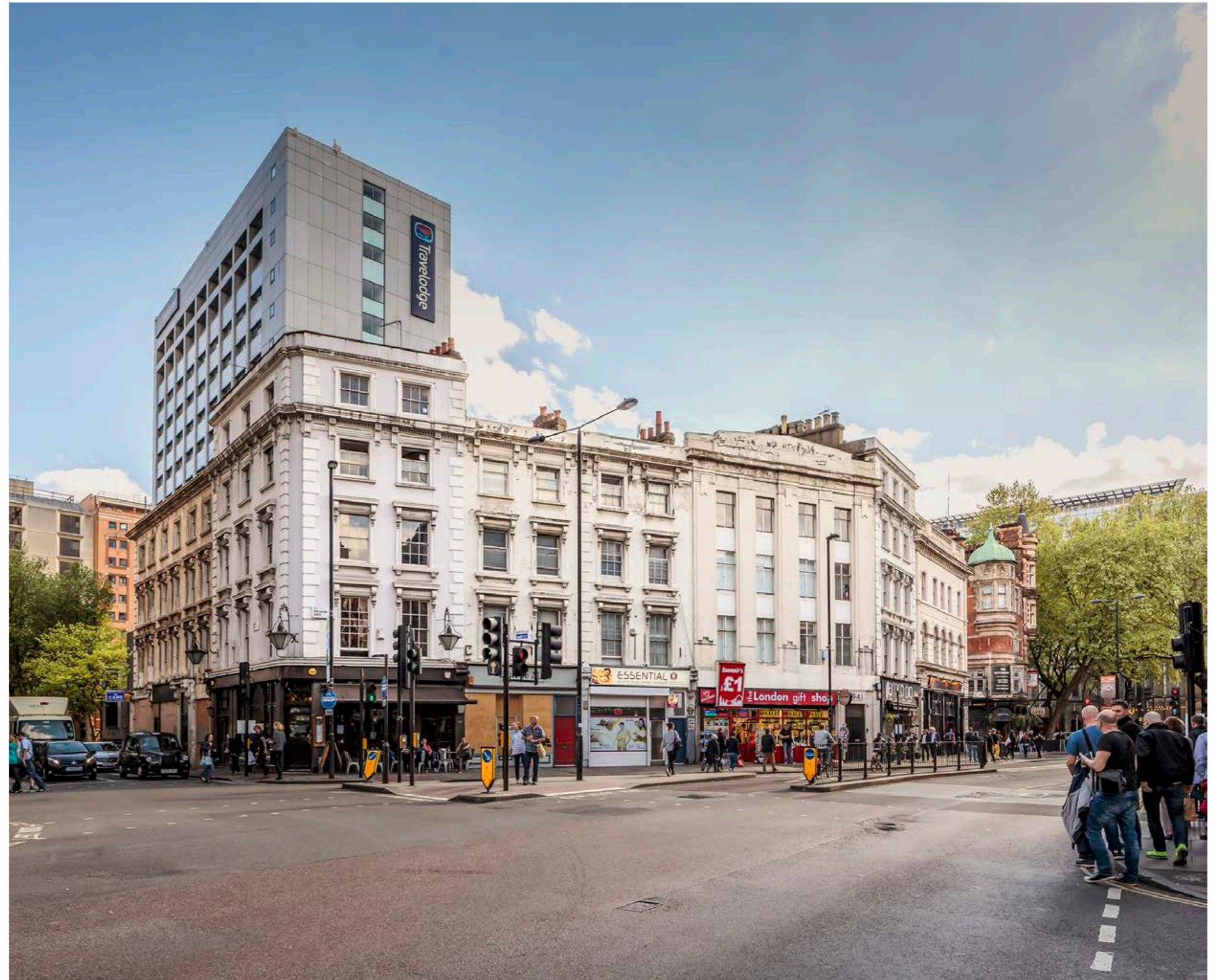
Existing view – Corner of Museum Street and New Oxford Street
