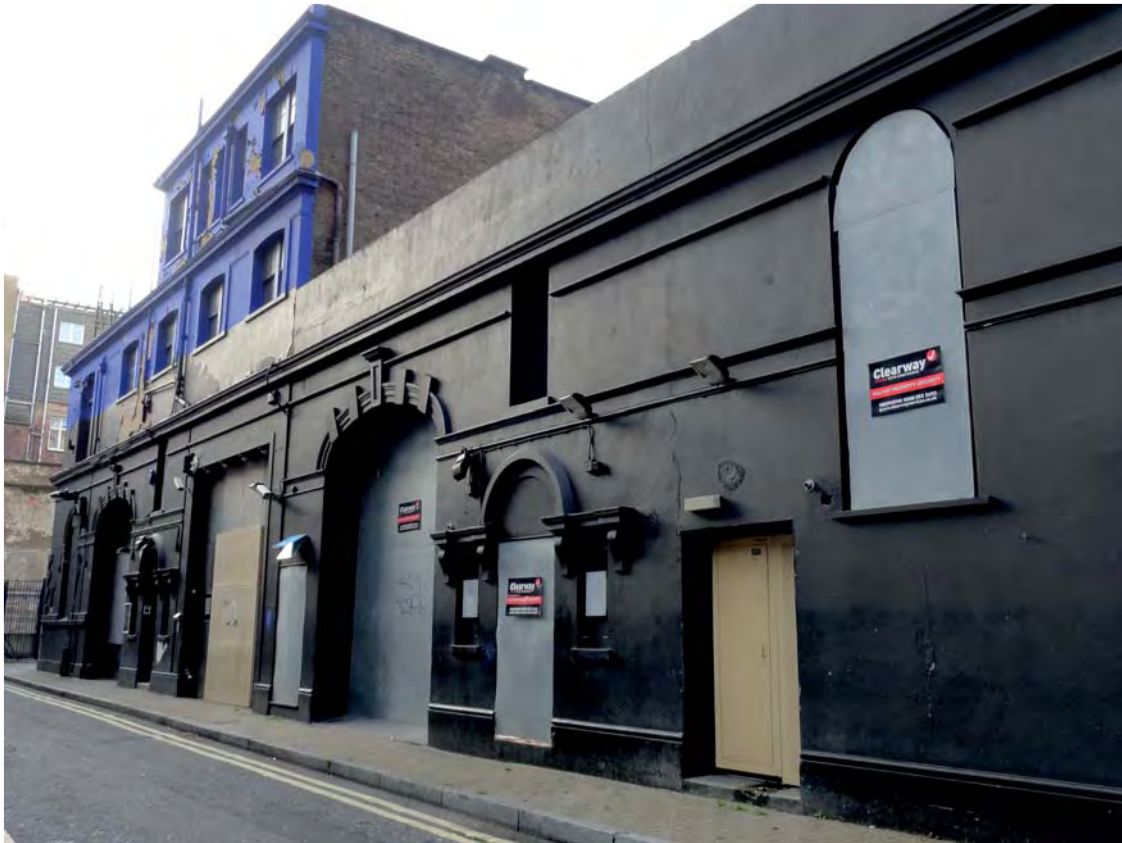
Fig 9 16a, 16b and 18 West Central Street façade; looking north-west (MOLA 2013)
