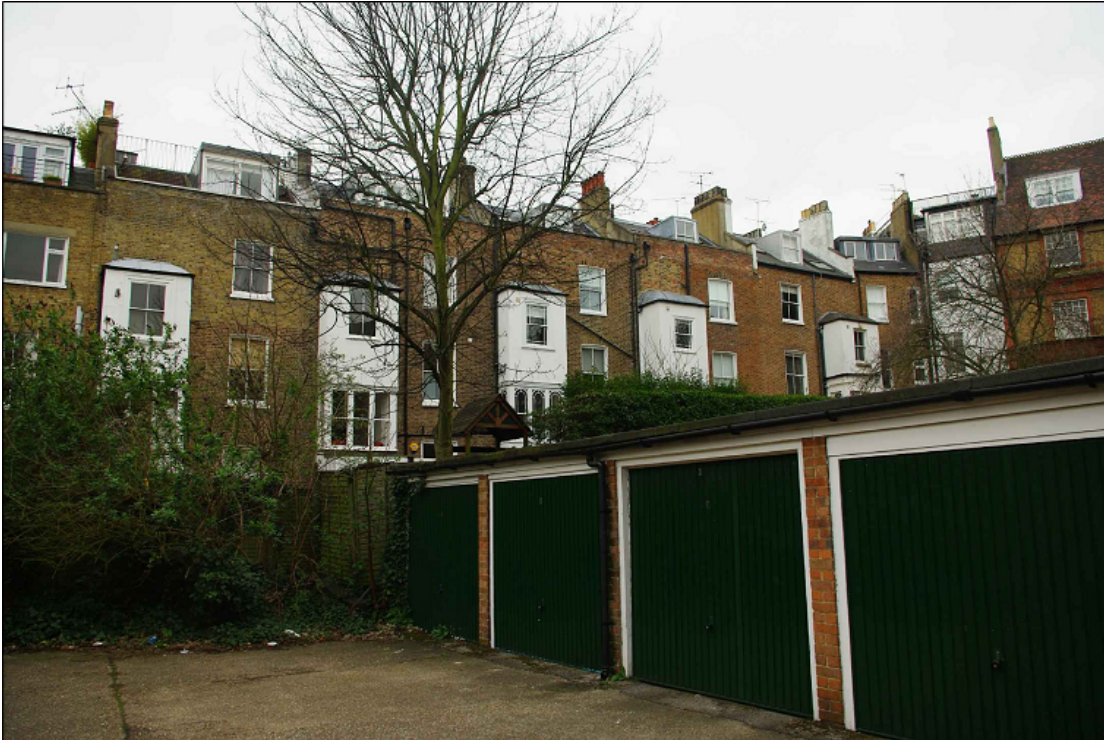
Photograph 1: View of existing garage block with T2 in background at 3 Belsize Place, London NW3 5AL
