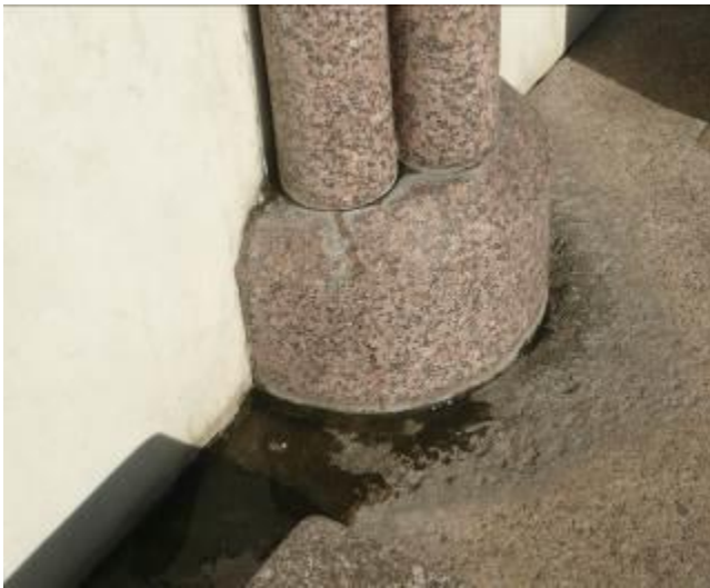
Active leaks though masonry on south side.
