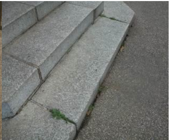
Weed growths on failing masonry joints
