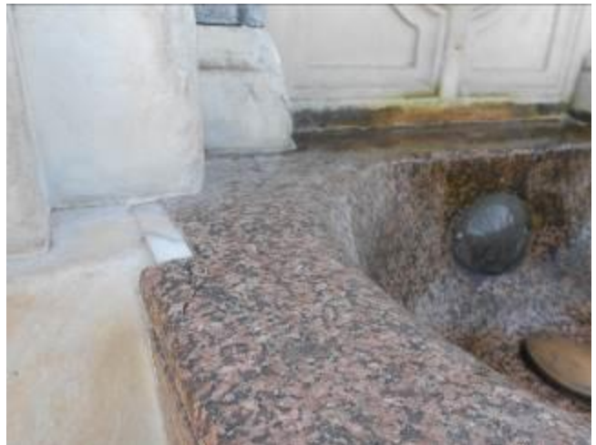
Uncontrolled overflow from fountain ponding on masonry
