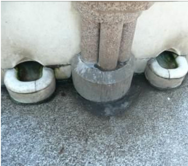
Leaks though masonry joints on north side.
