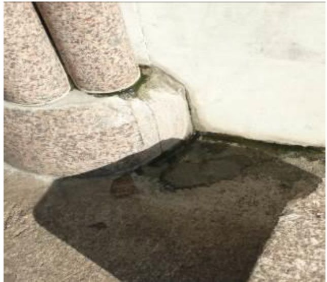
Active leaks though masonry on west side.
