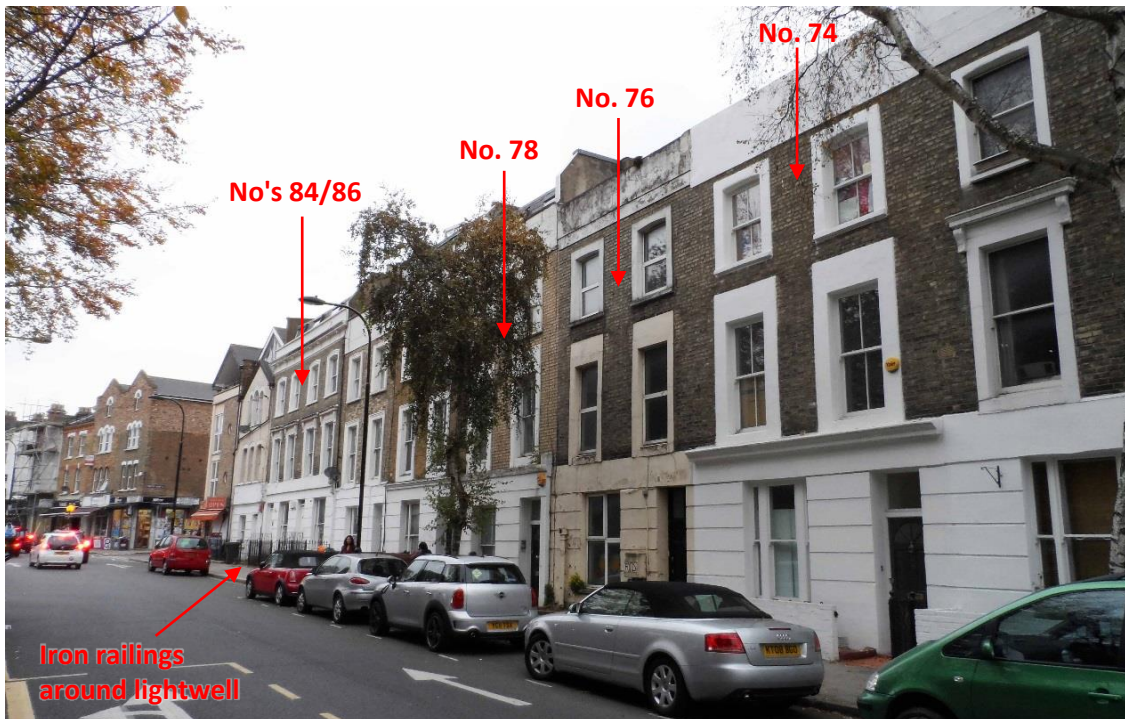
Photo 2: Front elevation (street scene) looking north-west. To the west of No.76, No's 84/86 Fleet Road have basements, with iron-railings around the front lightwells.
