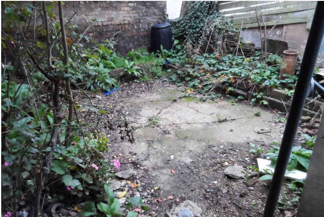
Photo 5: The rear garden is surfaced with paving slabs alongside the rear projection, and concrete beyond it, with a perimeter raised flower bed formed from 'railway sleepers' surrounding the rear part of the garden. The brick boundary wall between No's 74 & 76 is in poor condition.
