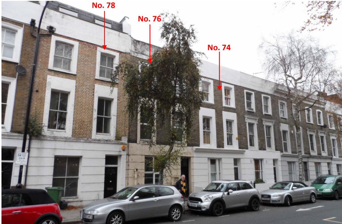
Photo 1: Front elevation (street scene) looking north-east. No.76 Fleet Road is a 3-storey, mid terrace house, situated on the north side of Fleet Road, between No's 78 and 74.
