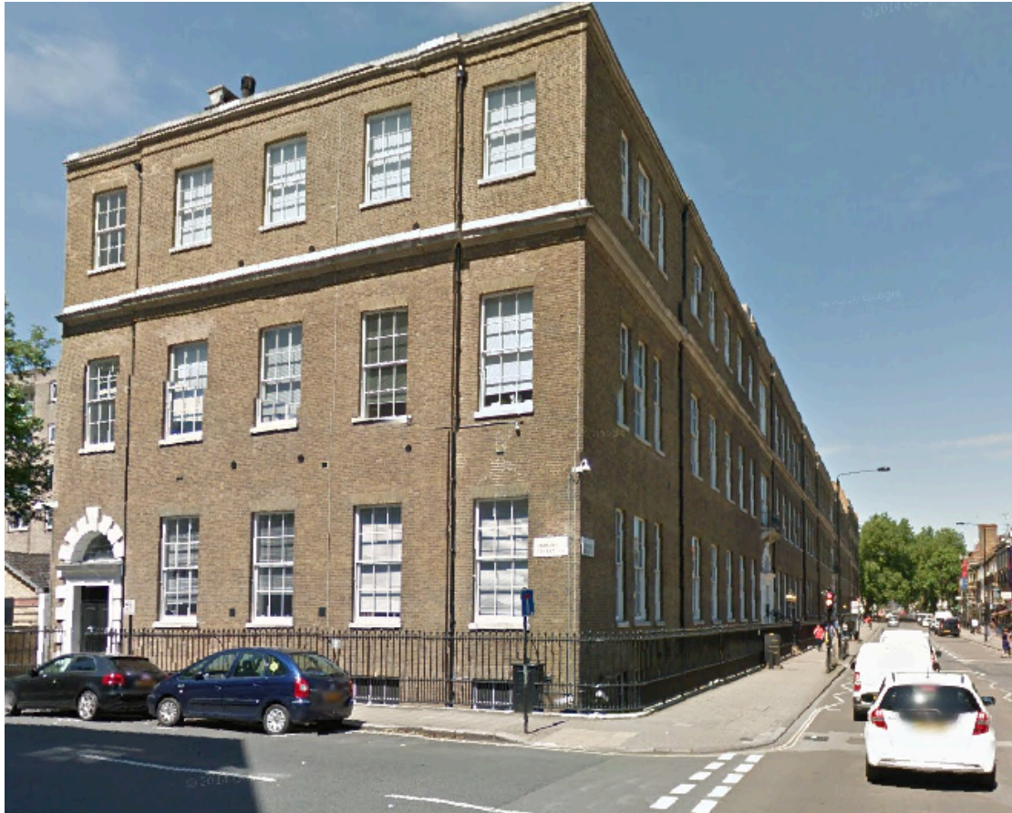
Fig. 2 view along Eversholt Street from south
