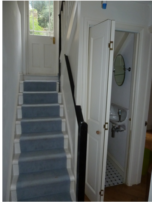
Original stair and door to rear garden.
