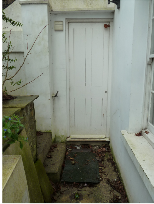
Door and front light well.
