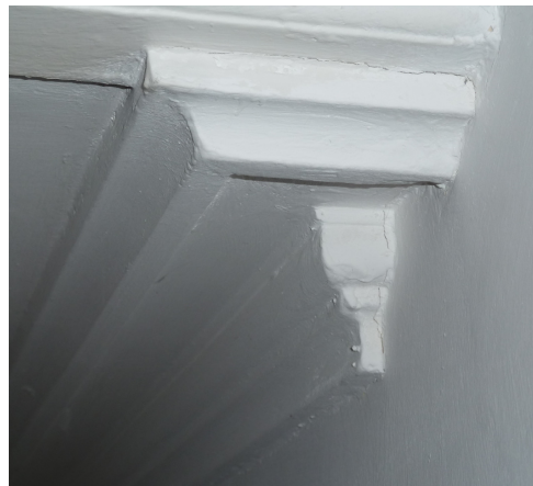
Existing cornice on ground floor.
