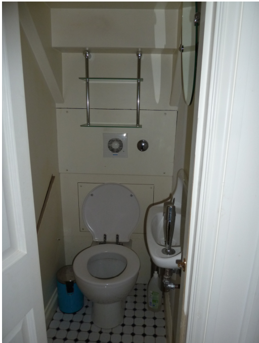
Existing cramped WC under the stair.
