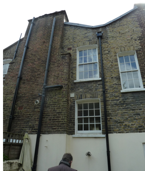
Rear of house and chimney breast.
