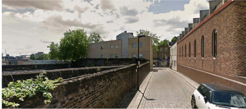
Fig. 3: Photograph of east elevation of host building.
