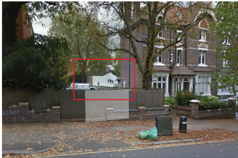
View of existing building from Fitzjohns Avenue
