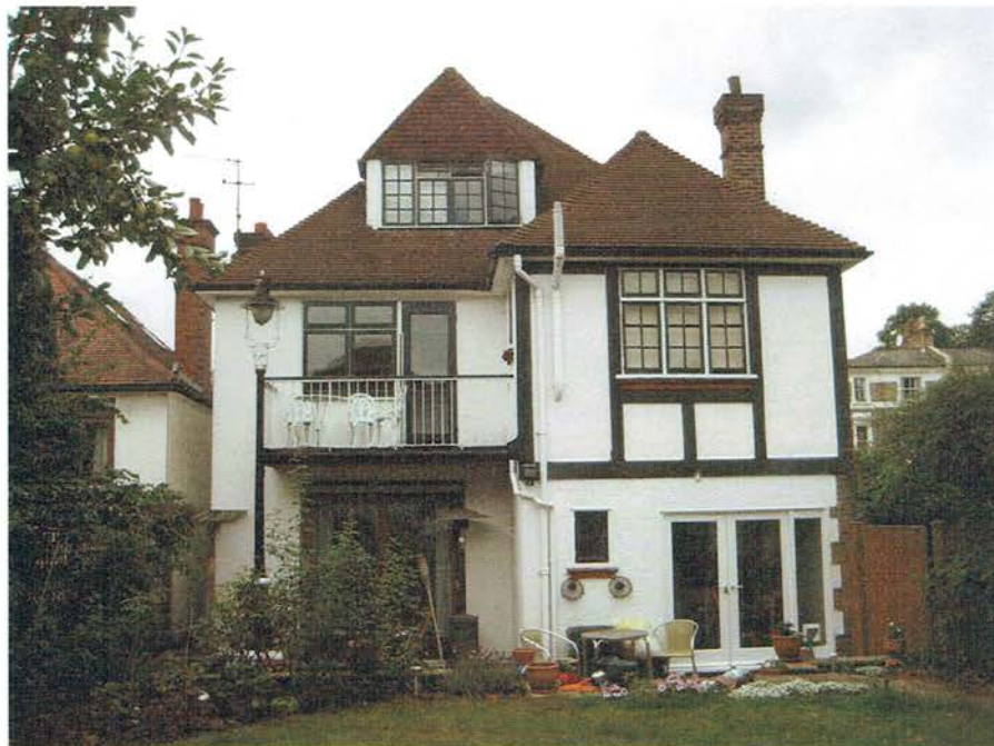
FIG 1 OLD FIRST FLOOR BALCONY/TERRACE TO REAR REMOVED (2013) TO ALLOW FOR NEW REAR EXTENSION
