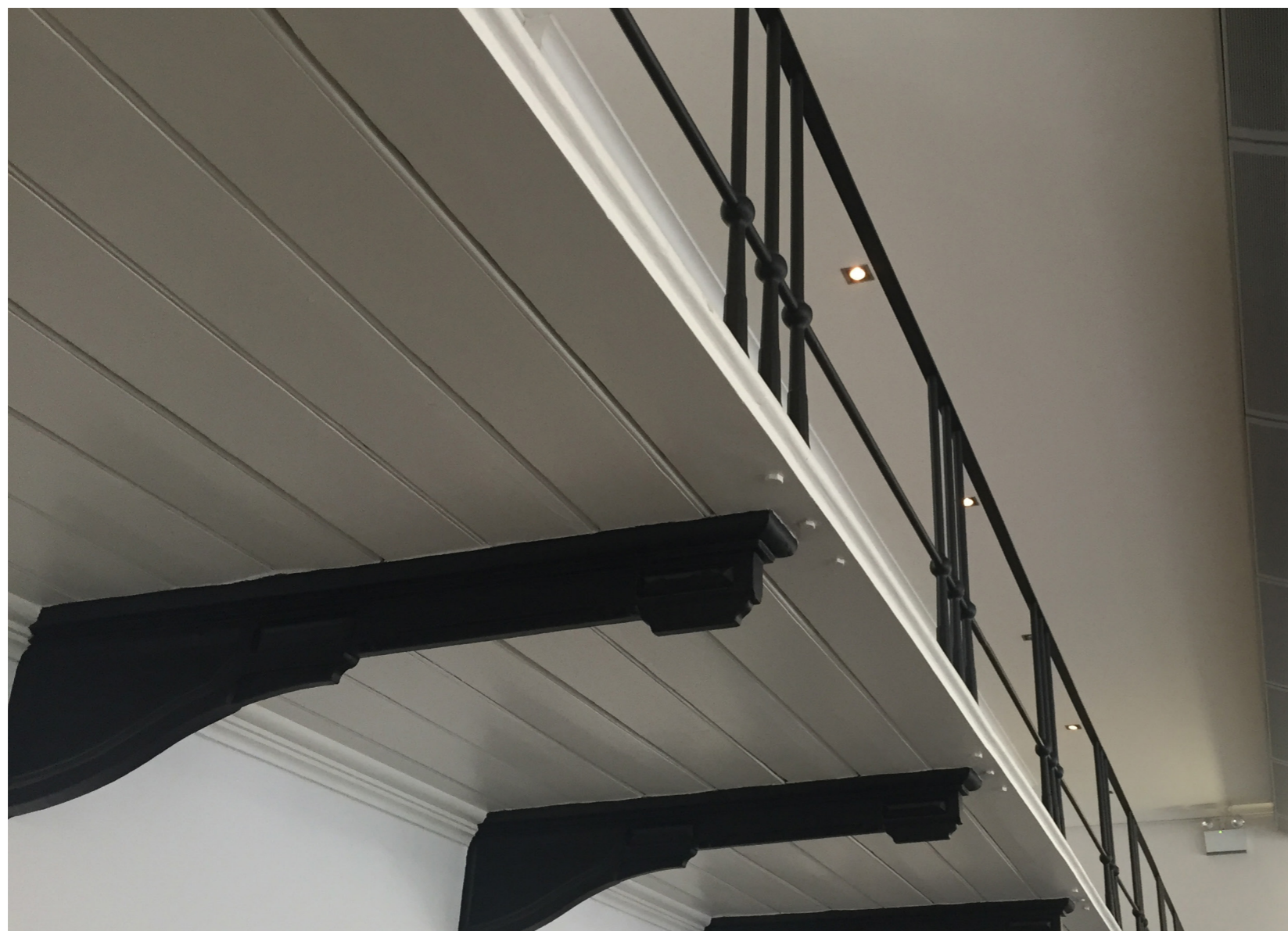
View of the historic mezzanine floors to the lower floors
