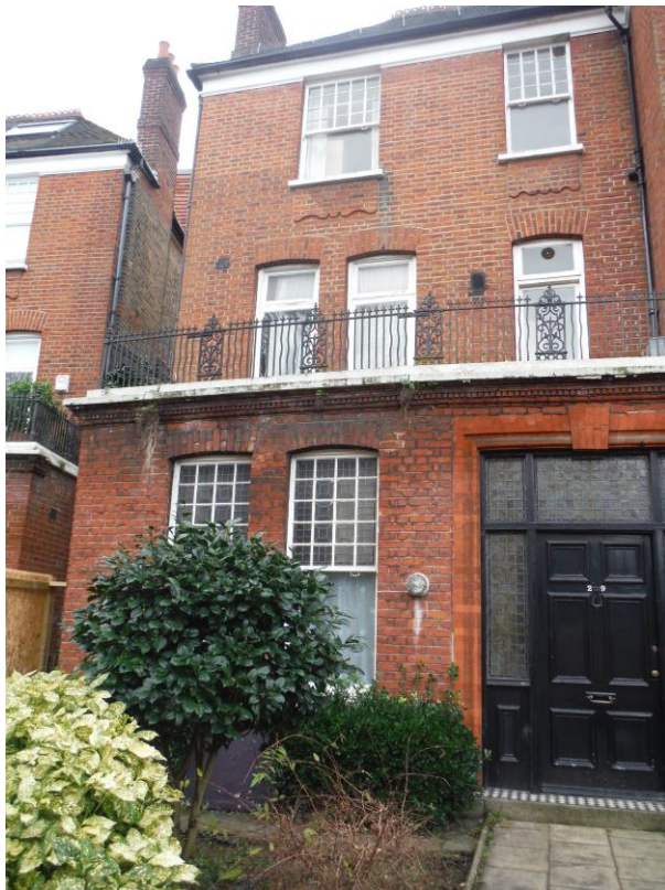
Front elevation of property, which would remain unaltered to the elevations. There would also be no change to the garden.
