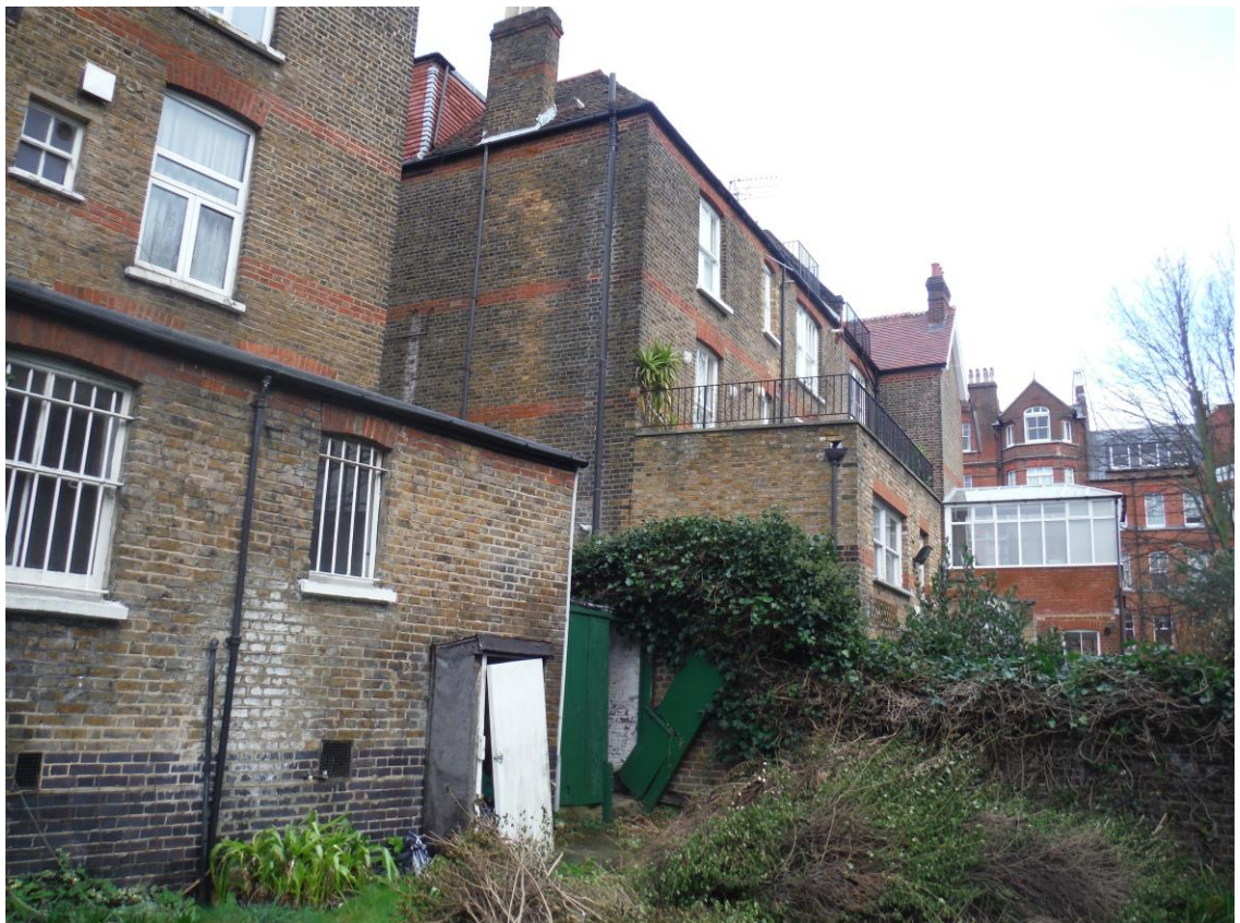
View of adjoining properties, showing extensive changes to the area
