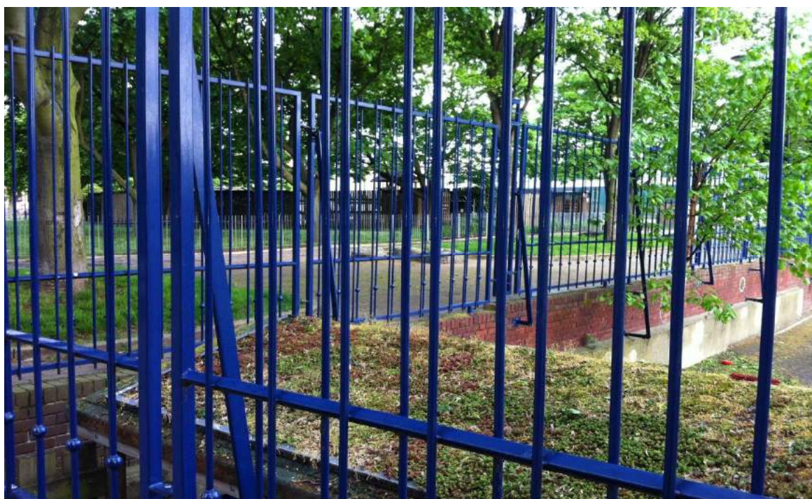
Figure 2: View looking north across Edith Neville Primary School (northern parcel of land) from Polygon Road
