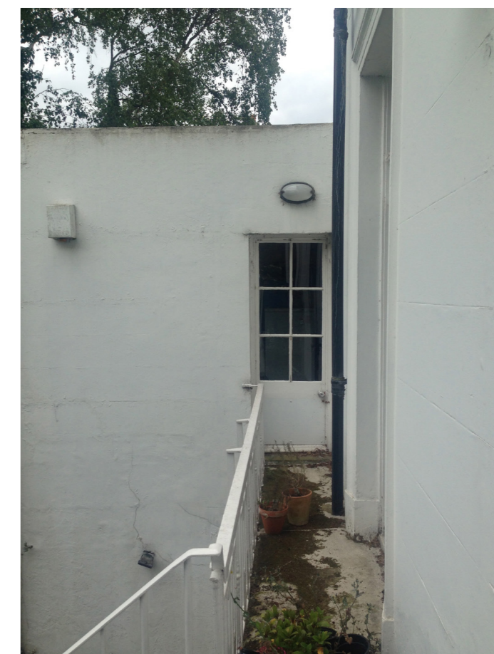
Image 07 - Existing balcony, upper ground level
