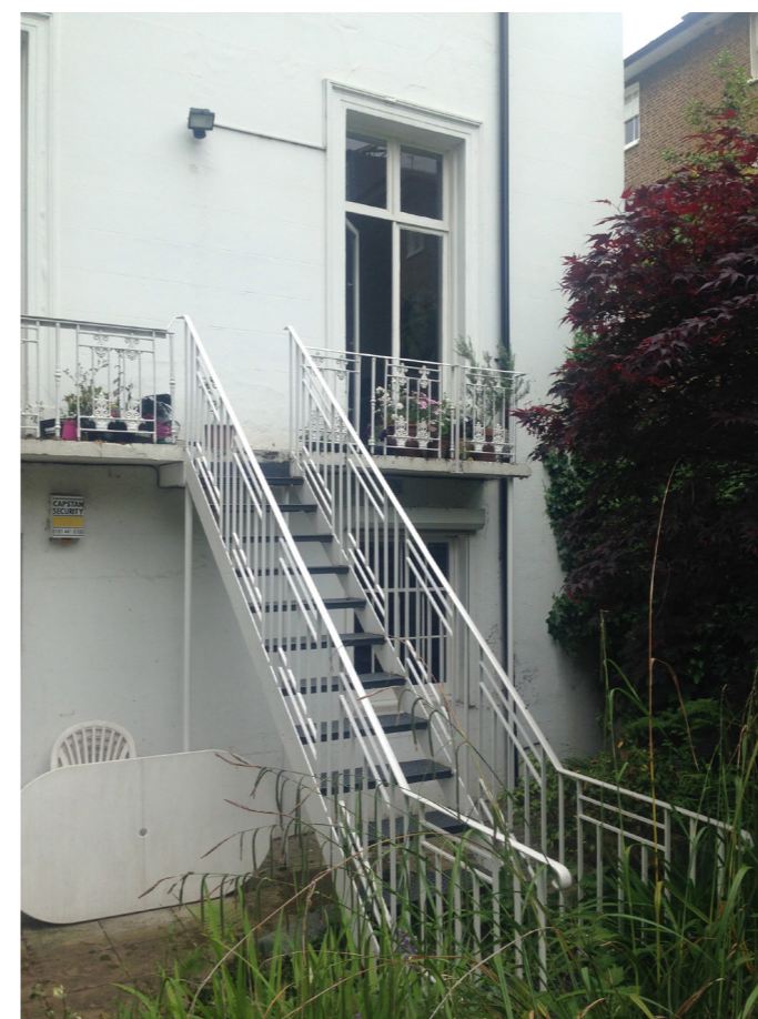
Image 06 - Existing stair, access from upper ground level to rear garden
