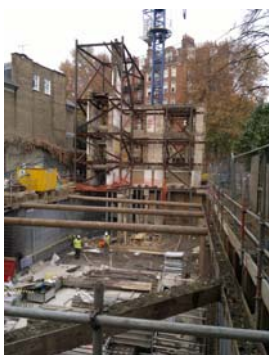
60 Addison Road W14 Facade retention over new basement
