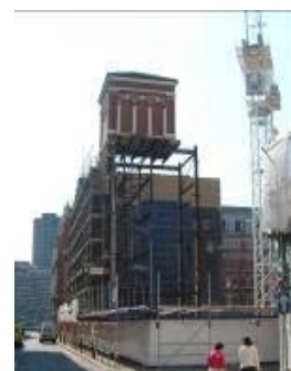
Whitefriars, London Facade & water tower retention prior to basement construction
