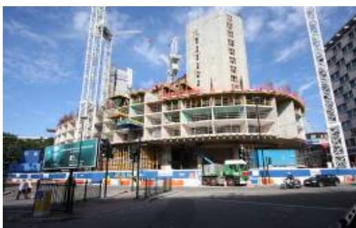
Westminster Park Plaza, London Construction of new luxury hotel by top-down method incorporating 4 basement levels
