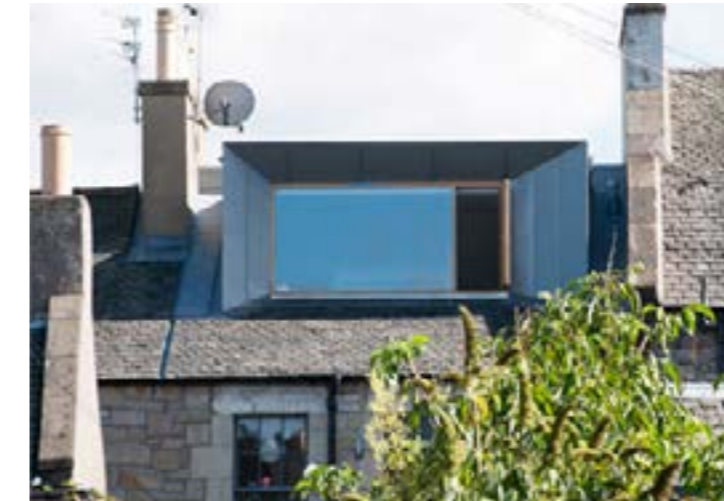
Contemporary dormer window showing crisp profiled dormer cheeks.
