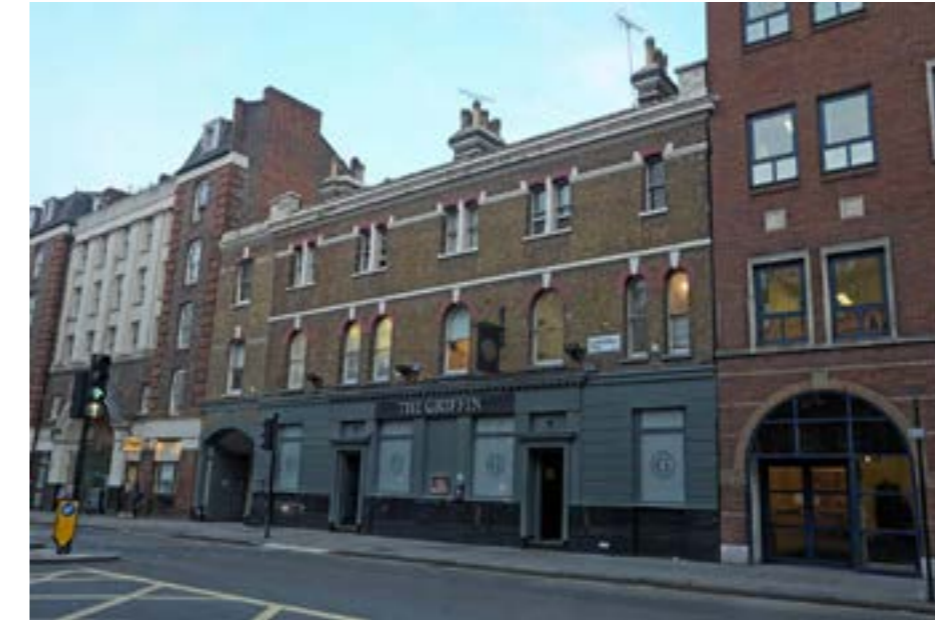
View looking West down Clerkenwell Road towards No. 125
