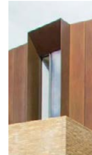
Profiled copper dormer window detail.
