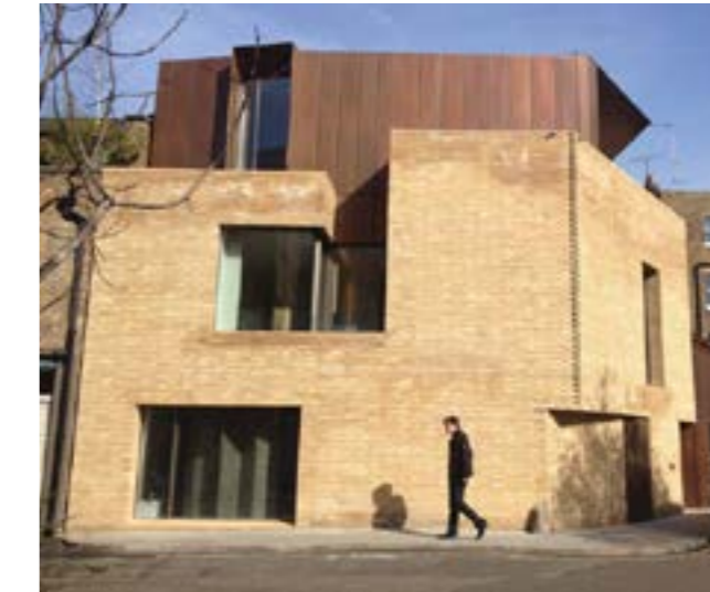
Bronze copper cladding of Leving House by Jamie Fobert Architects. (Located within Bloomsbury Conservation Area, Camden)
