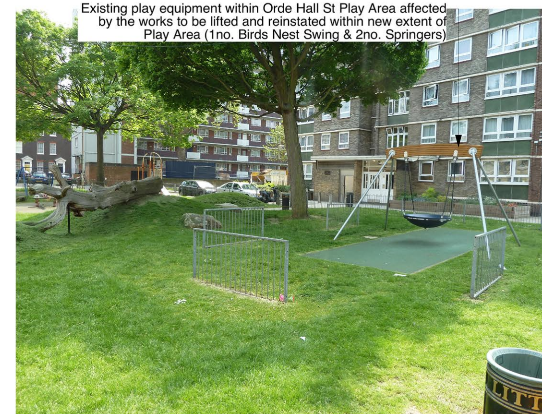
Image Of Existing Coloured EPDM Safety Surface (EPDM) Within Orde Hall Street Play Area (Exact Colour To Match Existing Safety Surface) Scale: 1:20 at A1
