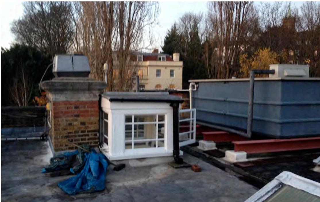
Roof lantern used for access [of later date than original building] with water tank behind – the proposals will demolish this small lantern to provide a safer access hatch, with a benefit to the original chimney.
