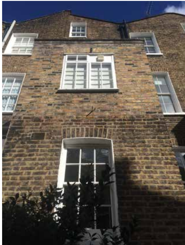
View of rear of building showing modern extension to closet wing.
