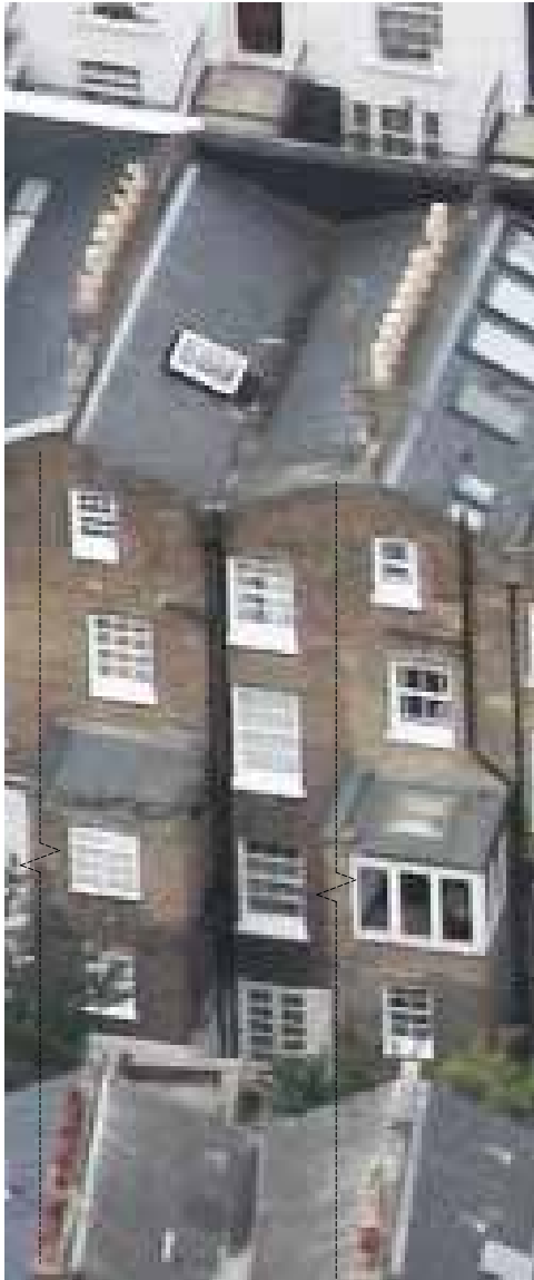
Rear elevation showing extensions to closet wing.
